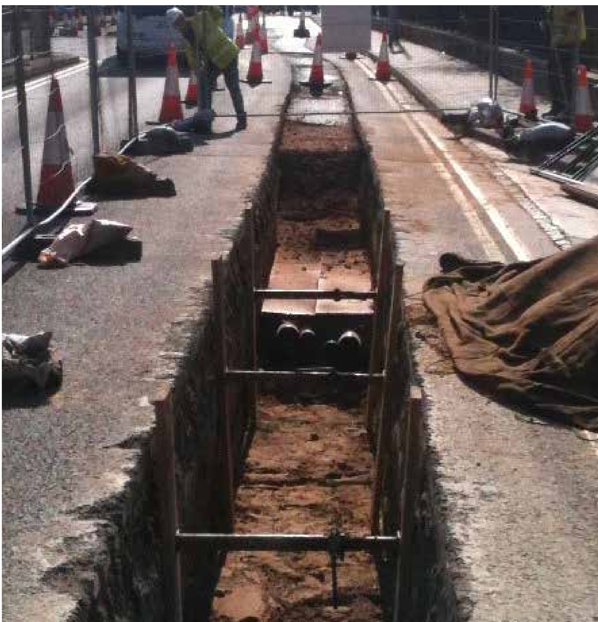
Indicative backfilled trench ducts (courtesy from Neary Construction)
